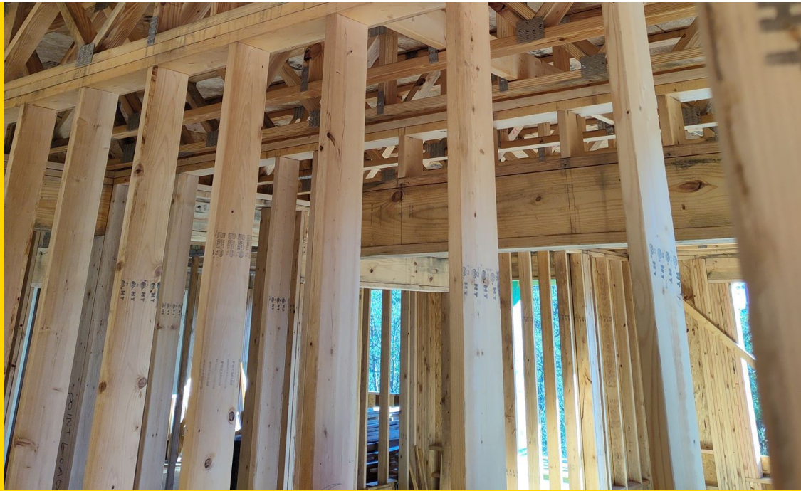
Interior photo of Prout Research Institute under construction
